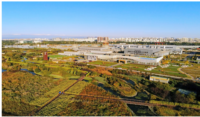
Aerial view of the wastewater treatment plant
